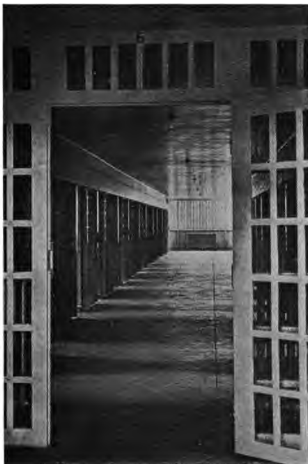
CELL BLOCK CORRIDOR
